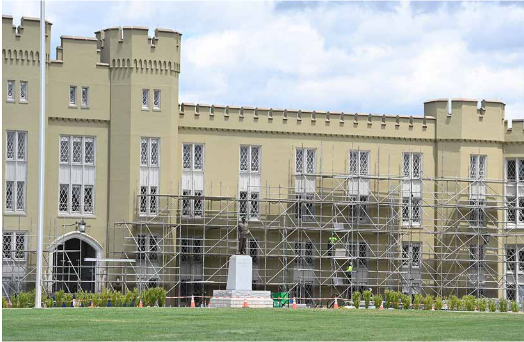
Scaffolding is put into place in front of New Barracks so workers can begin to replace barracks windows.—VMI Photo by Kelly Nye.
