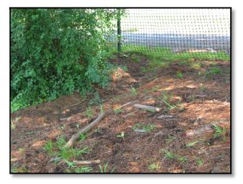
Virginia Military Institute Stormwater Master Plan The 'ditch' along the south side of the Woods Creek Trail captures runoff from the hillside to the north and has naturally created a drainage path under the safety fence, which ultimately discharges, and therefore creating erosion issues, down the embankment.
