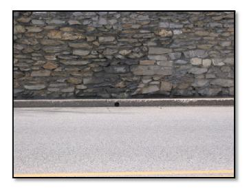
Additionally, the retaining walls, mortar-set field stone walls, are in good condition, except certain areas should be rebuilt with the existing stone by removing the old mortar and setting the original stones with new mortar. The drainage and weep hole system should be connected to a storm sewer system where possible.
