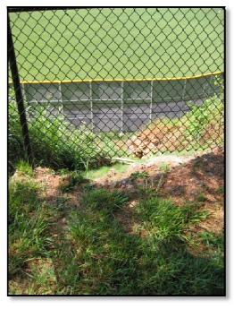
The embankment north of Gray-Minor Stadium is being eroded during significant storm events from runoff from the upstream watershed, which includes the Woods Creek Trail. The following photographs show the bank erosion back to the source along the Woods Creek Trail.
